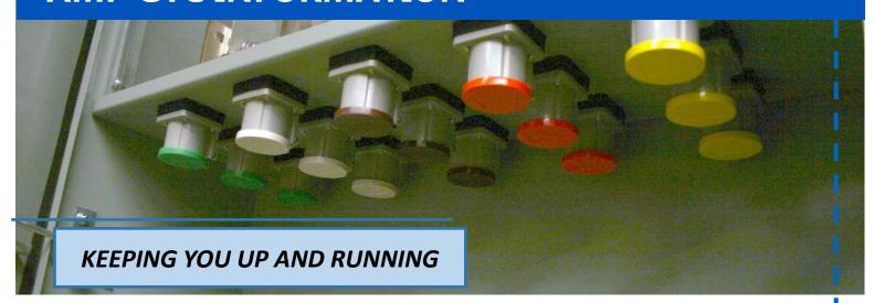
The American Midwest Power Generator Termination Cabinet (GTC) is specifically designed to be connected quickly and easily to a portable (mobile; roll up) generator.
