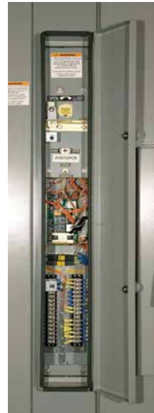
Figure 2. Hinged, gasketed cover protects motor operator from the environment and internal heater keeps air circulating to dry the interior.
