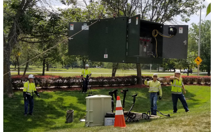
Figure 7. ISG-SD design allows for easy retrofit of existing air-insulating switchgear with no re-cabling or no new pad work needed.
