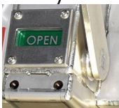
Open switch position indicator
