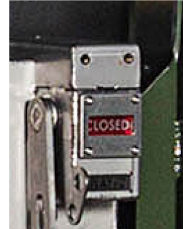
Motor operator provision and switch handle locking provisions
