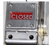
Closed switch position indicator
