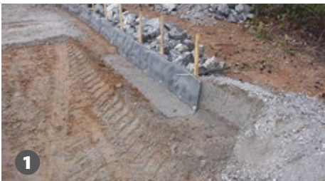
1 Water gate install to process water.
