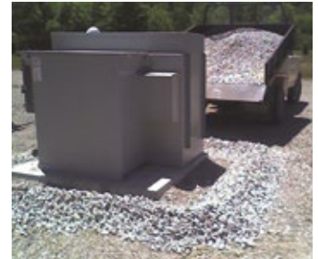
Pad mount for smaller containment.
