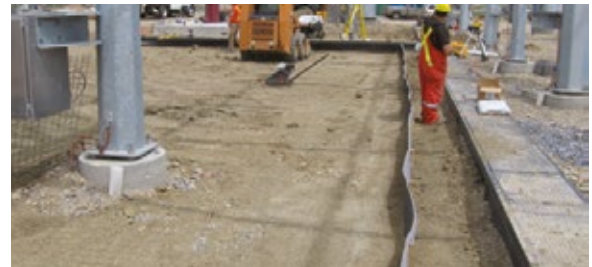
Site preparation and installation
