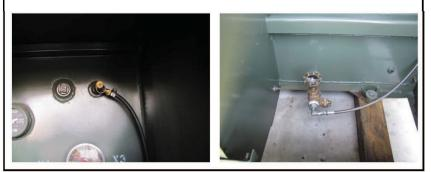
**STEP 8:** Zip tie the hose to the tank wall as desired.
