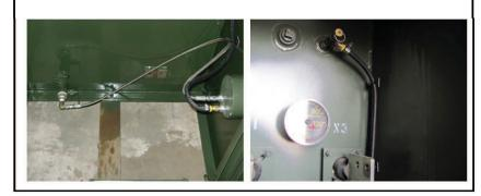
Always apply positive nitrogen or dry air blanket to transformer before pulling oil sample.
